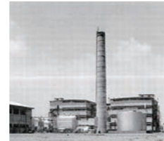
Tokai Production Plant at the completion of phase 1 construction
